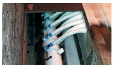
Plastic rink piping connections to the distribution and the collection mains (thermally insulated).
