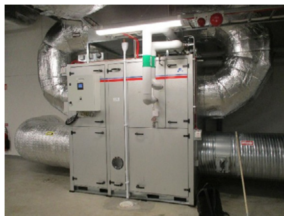
Figure 41. The working principle of a sorption type of dehumidifier [left] and unit [right].
