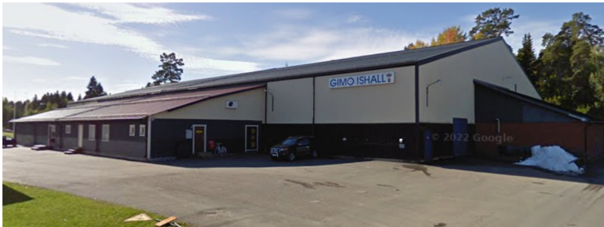
Figure 28. The first CO 2 primary refrigerant system in ice rink in Europe was installed in 2014 in Gimo, Sweden. Picture source: Google maps.
