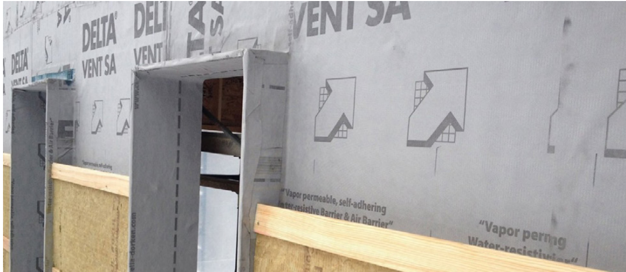
Figure 14. Vapour permeable Polyethylene self adhering air barrier [Delta Vent, 2019].
