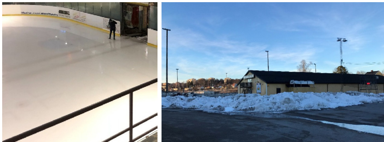
Figure 60. Issues often present by conventional resurfacing snow dump. On the left – tracks on ice due to resurfacer wheel dirt. On the right – snow accumulation outside the ice rink.
