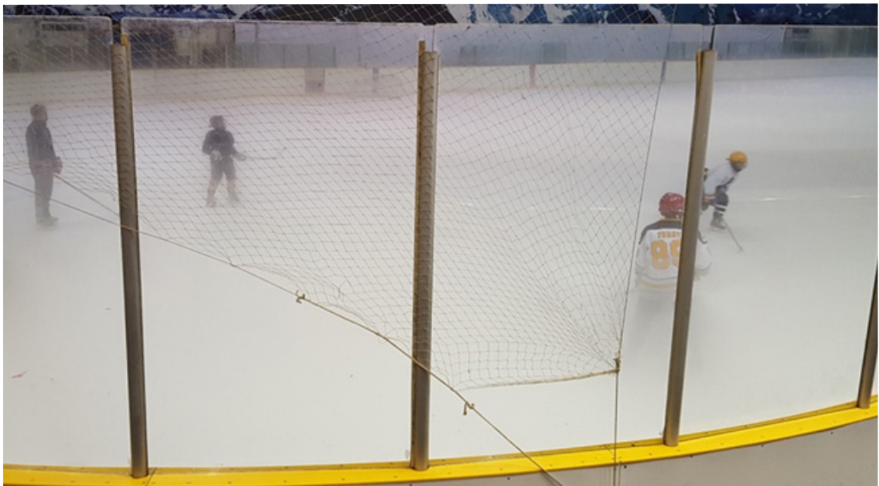
Figure 3. A well-functioning ice arena must be able to handle the complex heat loads and moisture loads that come along with this specific environment. In this picture they are not well managed, causing foggy conditions.
